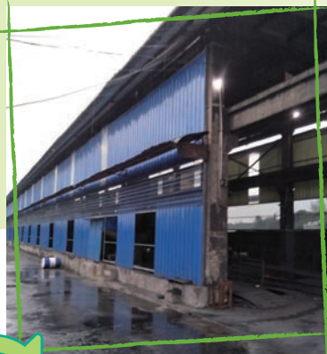
Train unloading operation workshop and coal conveyor belts are sealed at Yichang Port
